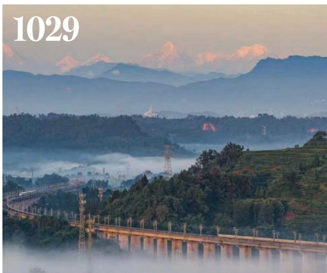
The eastern segment of the Sichuan–Tibet Railway traverses a mountainous region characterized by complex hydrogeology and environmentally sensitive terrain.
